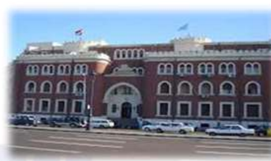
ALEXANDRIA UNIVERSITY ADMINISTRATION BUILDING
